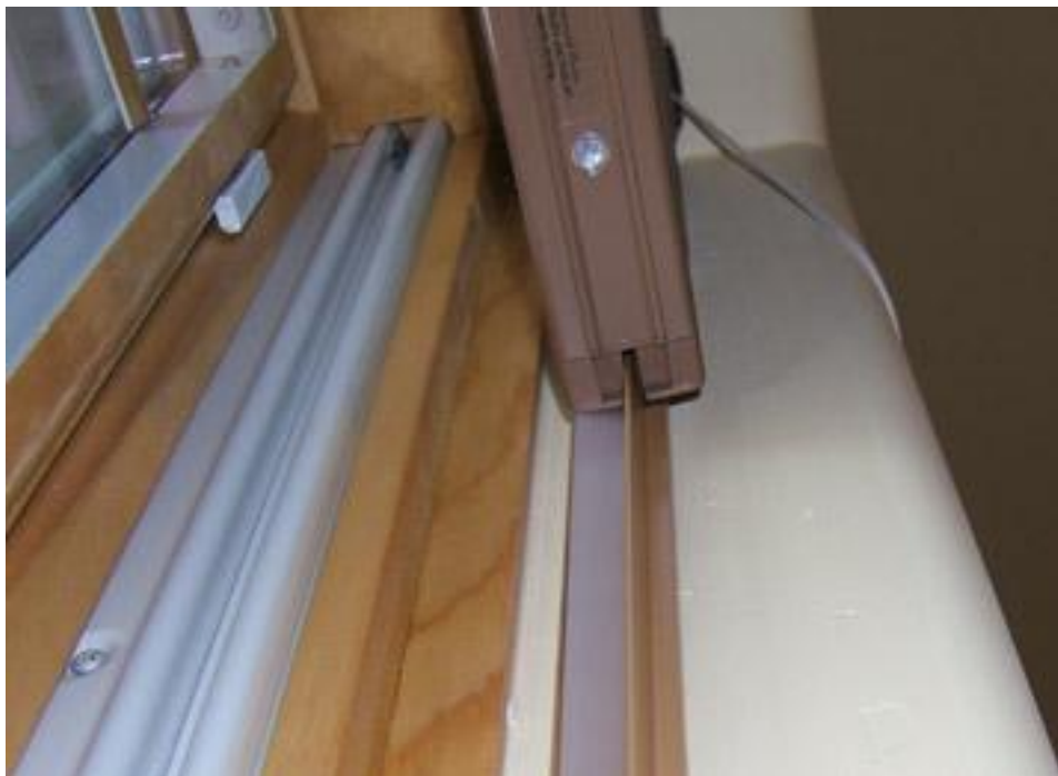
Figure 3. ComforTrack™ Plus Shades with Side Seals in Place.
